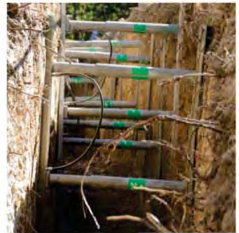
Trench excavations are a common tool used by geologists when evaluating potential geologic hazards, such as landslides or earthquake faults. Alan Hynes Construction performs trench excavations for Murray Engineers—a leading geotechnical firm in the Bay Area—when homeowners are evaluating whether a piece of land is suitable for building.
